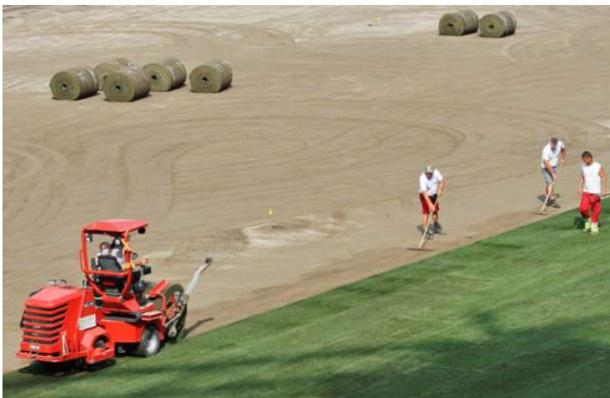
Sod laying - MIXTO SYSTEM
